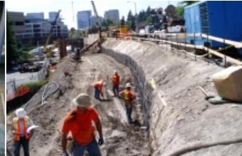
This temporary soil-nail retaining wall, shown during construction, is one of several installed.
