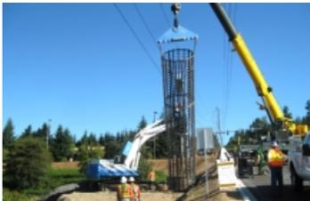
GeoEngineers monitors the lowering of the rebar cage into a drilled shaft.
