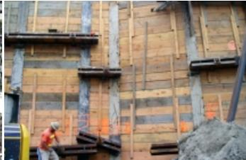
Tie-back walls provide temporary shoring and underpinning of an existing bridge.
