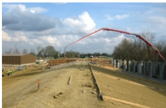
Constructing the elevated roadway over the levee
