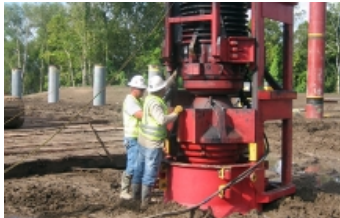
Piles anchoring barges were driven with large pile-driving equipment.
