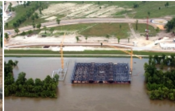
Aerial view of barges during high water before the casino was built atop them. © Aero Photo
