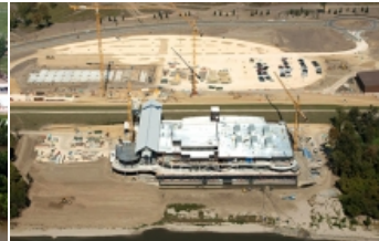
The casino was built on top of the floating barges. © Aero Photo
