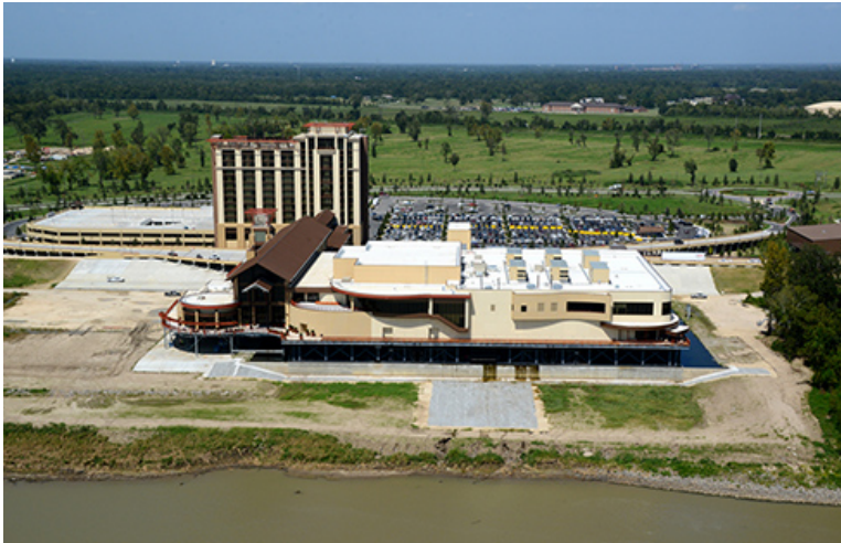
The completed floating L'Auberge casino, hotel and parking areas. © Aero Photo
