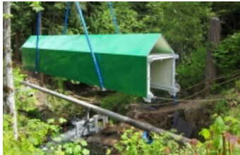
Lowering the protective truss over the pipe
