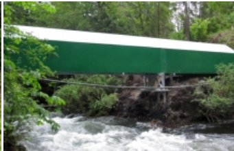
Truss after installation
