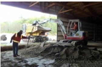
The contaminated soil and concrete floor inside the hangar building were safely removed without damaging the building.
