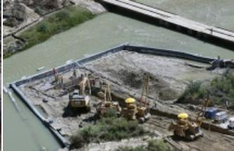
Side booms lowering the pipeline into the trench within the diverted river channel
