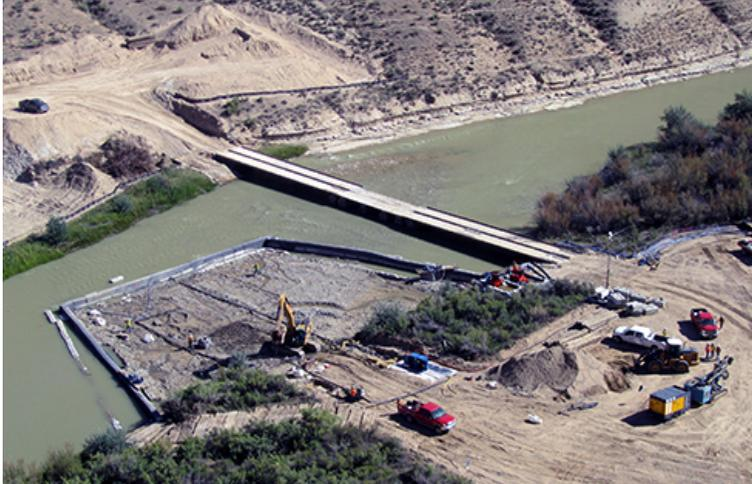
White River crossing site after temporary bridge and phase 1 diversion were installed
